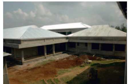
The roofed buildings of the male and female wards, July 2011
