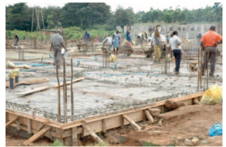
The Ward early phase, June 2010 – the foundations and ground floor in place
